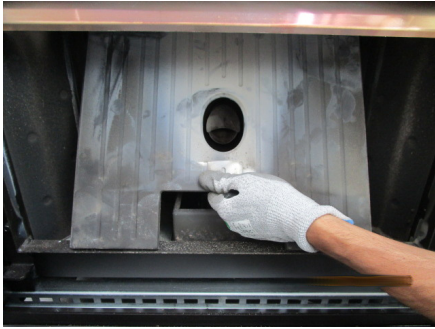
Fig. 39 - Central cast iron removal
